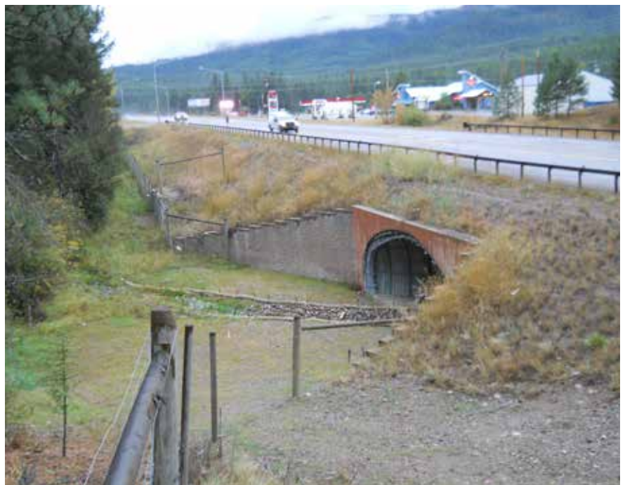
Fencing and tunnel guiding wildlife passage under Highway 93 on the Flathead Reservation. Photo by the Montana Department of Transportation
