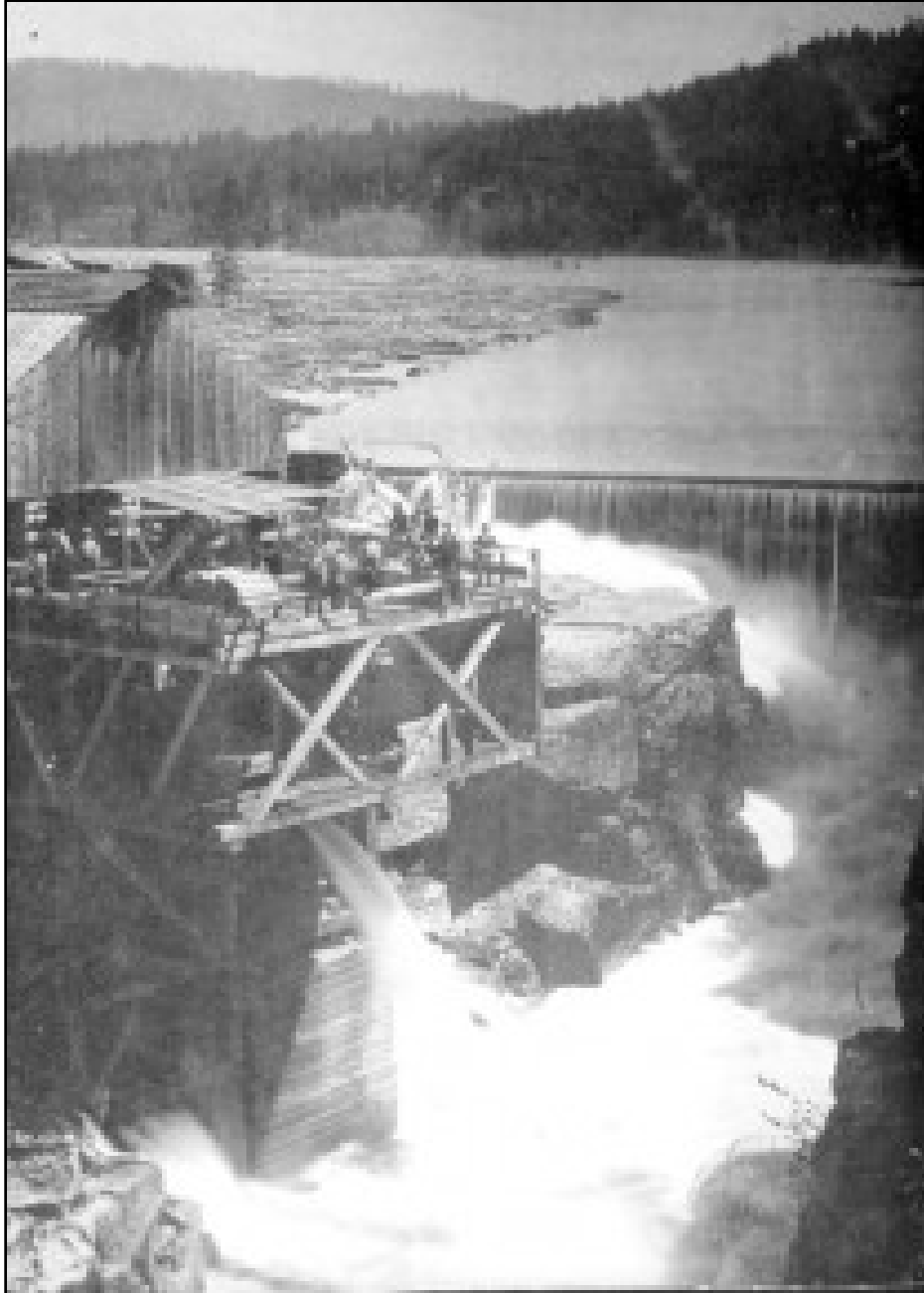
Figure 17. First lumber mill at Post Falls, Idaho where a 20-foot-high timber crib dam was erected to divert flow to the sawmill, ca. 1900.
