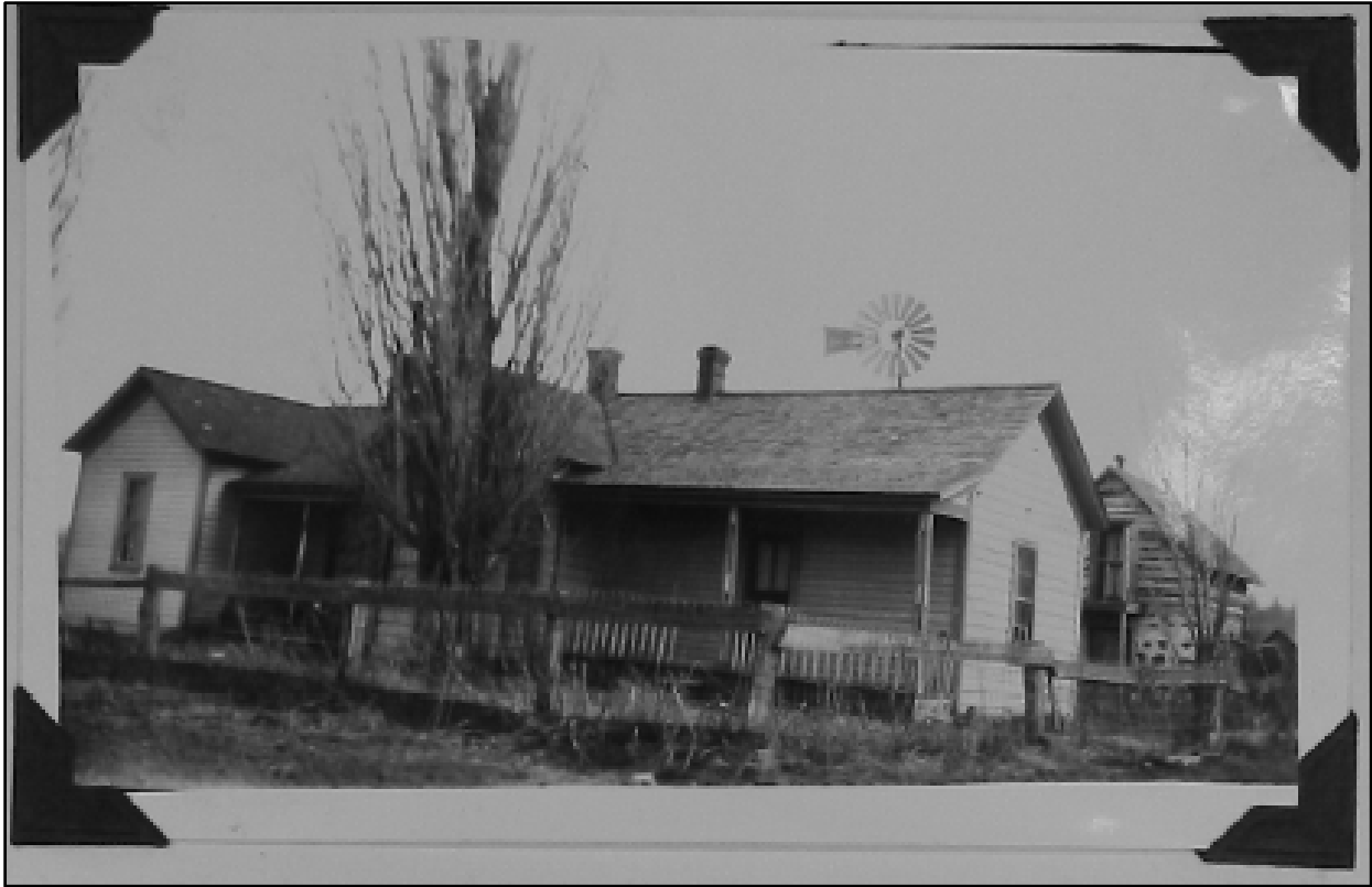
Figure 27. 1929 Photograph of the home of John Peone, Indian Allotment No. 638, whose water supply came from a well pumped with wind power.
